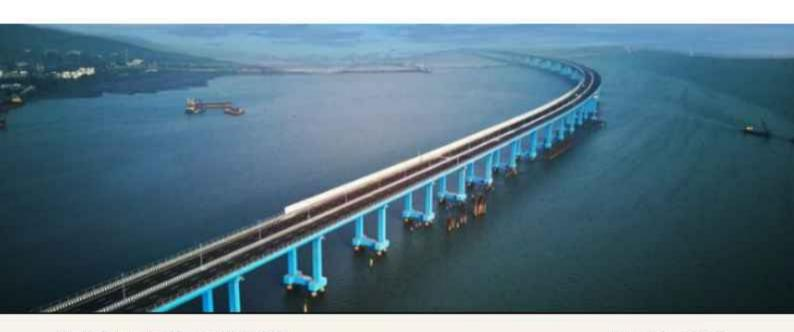
The orthotropic deck components were assembled at Karanja Port in Uran after being manufactured in Taiwan, Vietnam, Myanmar, and Japan. Each deck took roughly three days to erect after being transported by barge to the building site. The deck was loaded onto the barge using a self-propelled transporter that was programmed, and it was installed on the bridge using computer-controlled jacks that operated within a precise 5 mm band.
