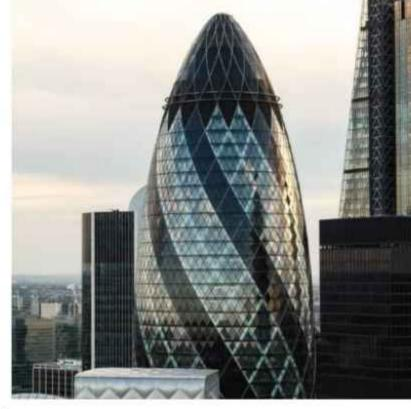
Double skin facades are Technological Marvel Inspired by Nature and are aptly named for their two-layer structure, are rapidly gaining popularity in the architectural world. These ingenious systems, consisting of two glass skins separated by an air cavity, offer a unique blend of aesthetics, sustainability, and adaptability.
